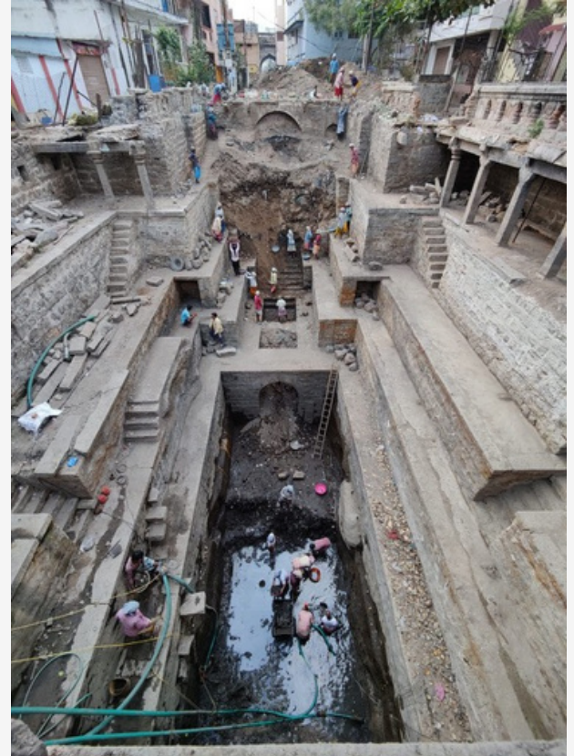
Bansilalpet stepwell of Telangana during restoration
