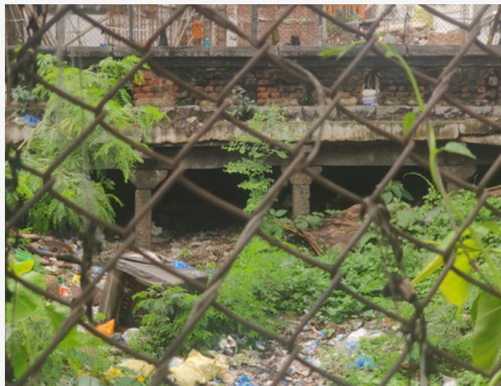
A section of bansilalpet before restoration
